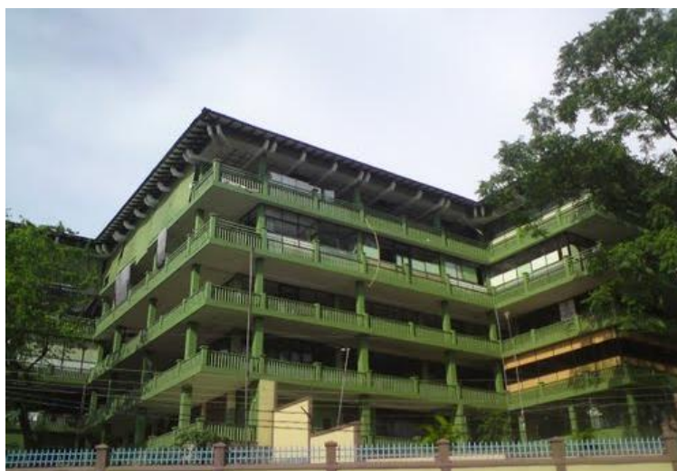
North Colombo Teaching Hospital - Ragama
